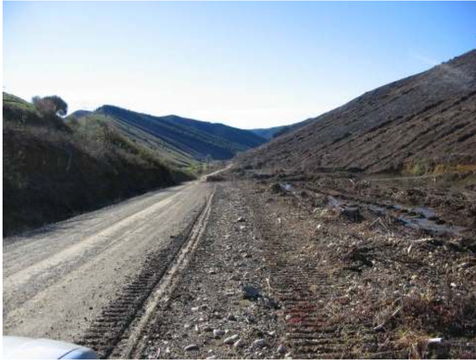
The present access road descending into Rabbit Gully, looking north
